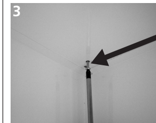
3 Blechschraube 4.2 x 13 Self-tapping screw 4.2 x 13
